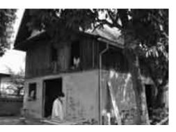
The walls of this old house were originally built using woven bamboo strips, finished with a lime-based plaster. But the house is being restored using cement instead of traditional plaster, compromising both the durability and heritage value of the building. (*Photo: Rik Ponne*)
