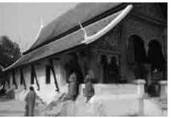
These monks have applied concrete and modern paint to the exterior of this temple and are applying gold paint to the columns instead of using traditional gilding techniques. Such renovation work compromises the durability of the building and decreases the heritage value of the site. (Photo: Rik Ponne)
