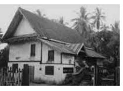
The damaged areas of the plaster walls of this building have been repaired with concrete, which apart from being aesthetically unappealing, diminishes the building's heritage value. (*Photo: Montira Horayangura Unakul*)
